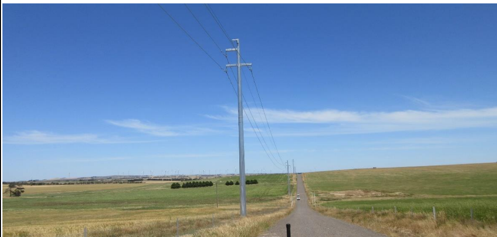
Plate 4.2 – Pole structures south of North Transition Station
