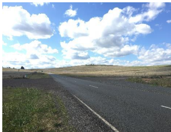
Plate 5. Intersection widening extent at Eurambeen-Streatham Road (A, Taylor. 9 April 2020).
